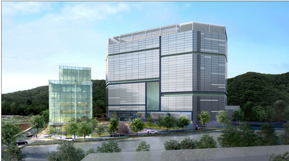
Figure 1 | Front view of Empyrium Digital's KR1 data center in Korea
